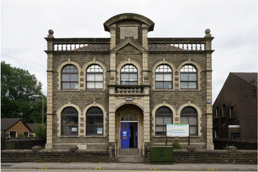
Taibach Library. One of the places where Mass was offered before the parish had a church of its own.
